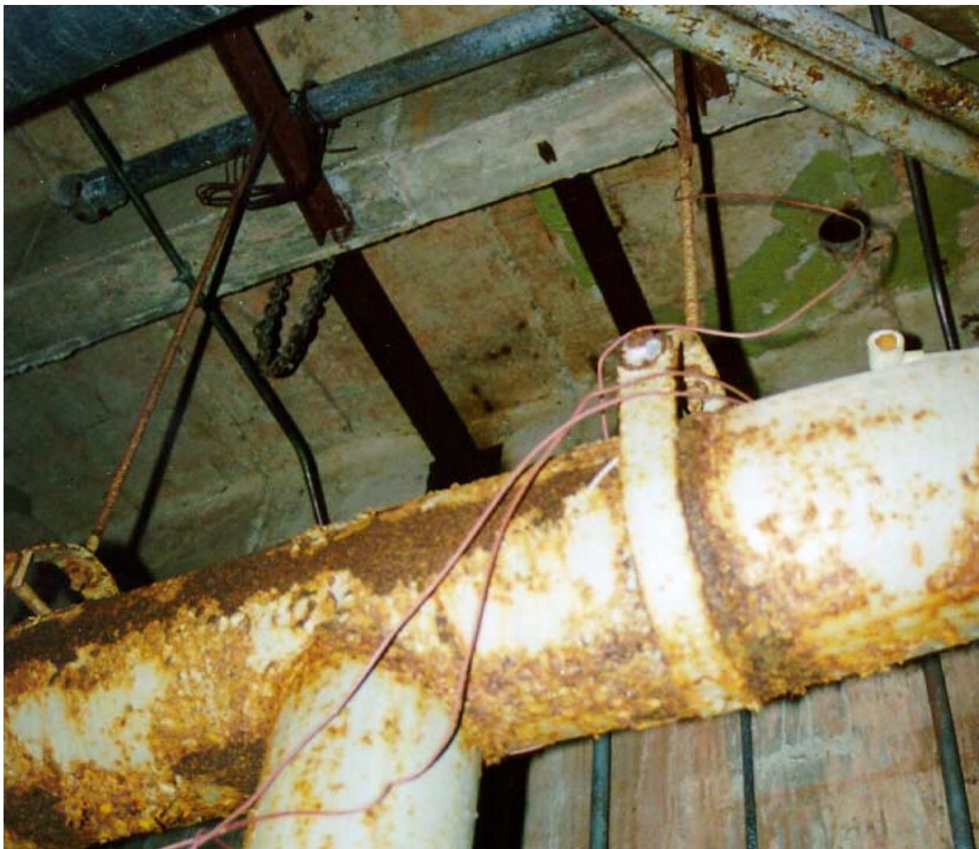
Improper bond to water pipe
