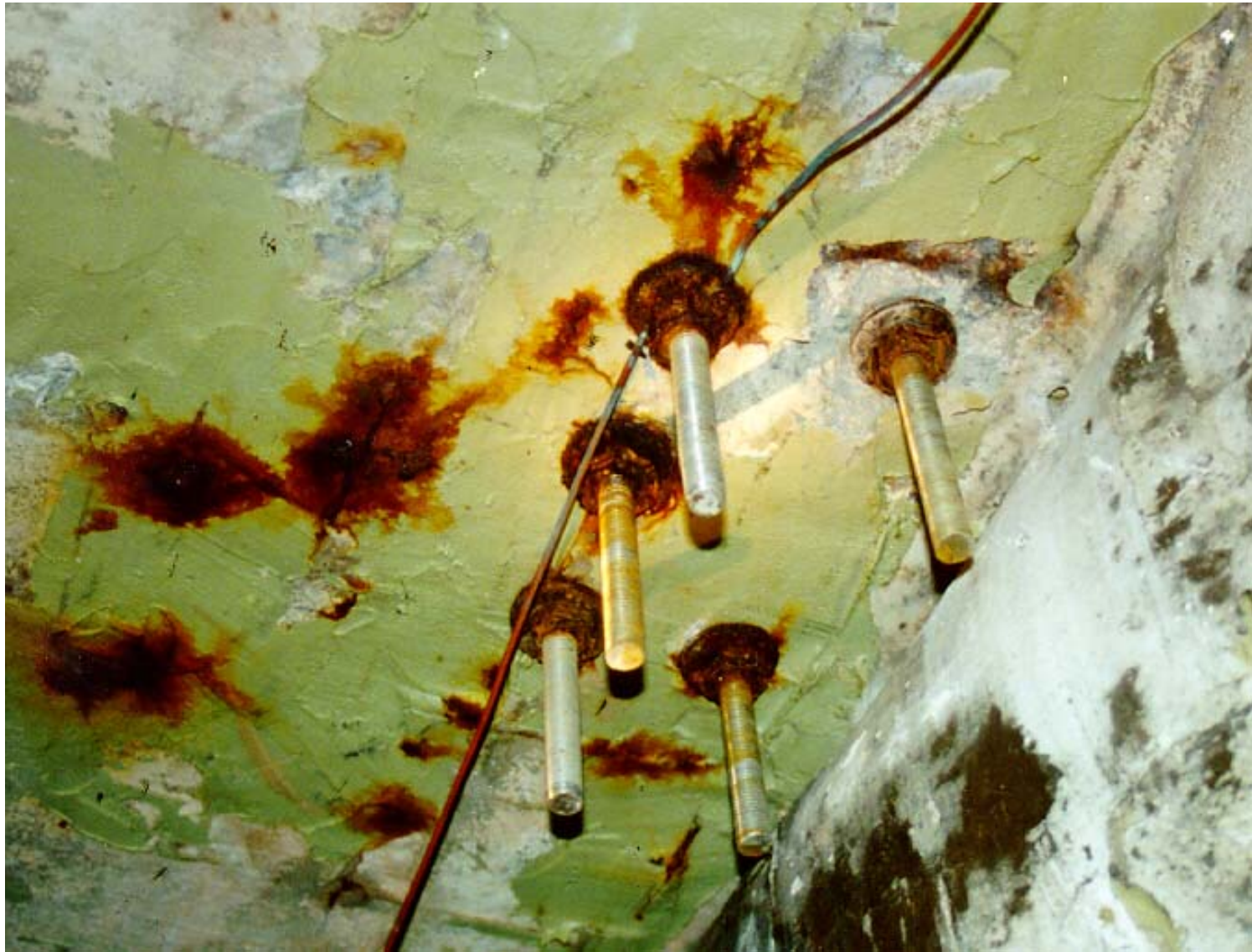
Improper bond to lifeguard stand
